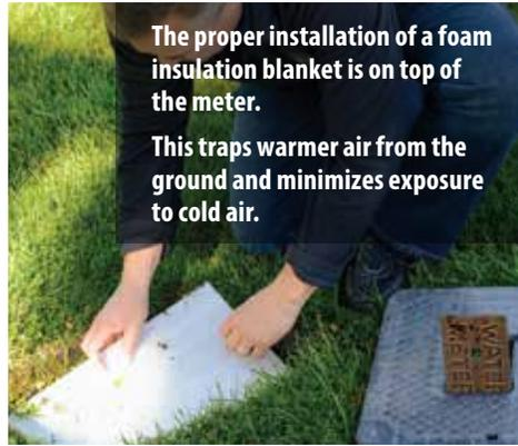
The proper installation of a foam insulation blanket is on top of the meter.
